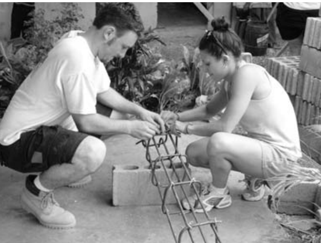
■ Sophomore Erik Weber and Marni Rakes '04 prepare to reinforce a column for the construction of a comfort room for an elementary school on Mactan Island.
